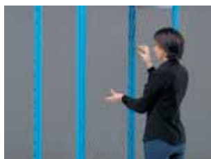
Assembling the mesh panel
