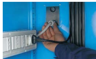
Adjust the external length of the power cable by unscrewing the relative cable holder. The dual protection power cable is 3 metres long.
